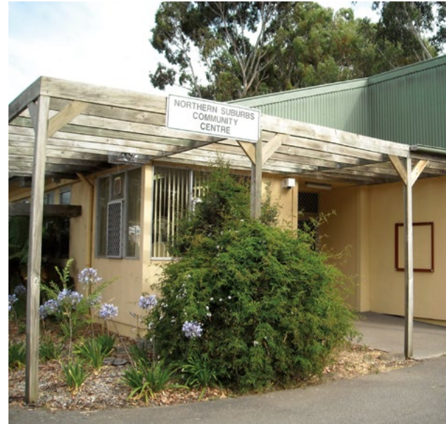
Northern Suburbs Community Centre Inc, Rocherlea site
